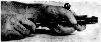
FIGURE 46. DRAWING COCKING PIECE BACK.
